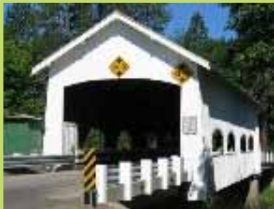
Rochester Cover Bridge
